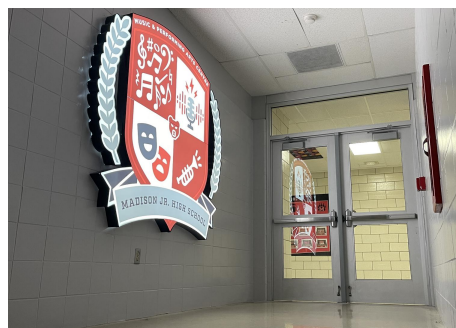
At left, the renovated entry hallway looking out from the classrooms.
